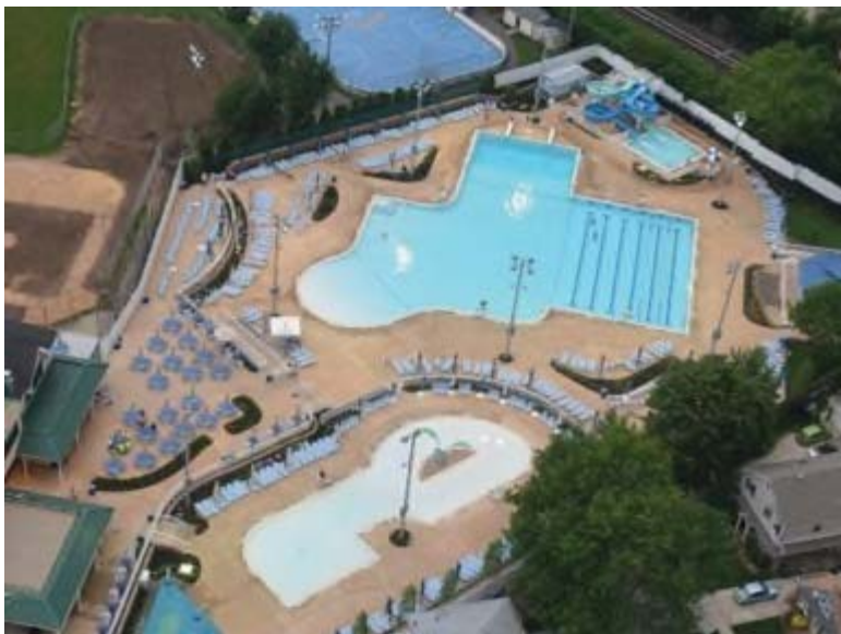
View of Floral Park Recreational Center, with Main Line in background. (source: https://www.shotcrete.com/what-we-do/pools-and-water-features/floral-park-rec-center/ )
