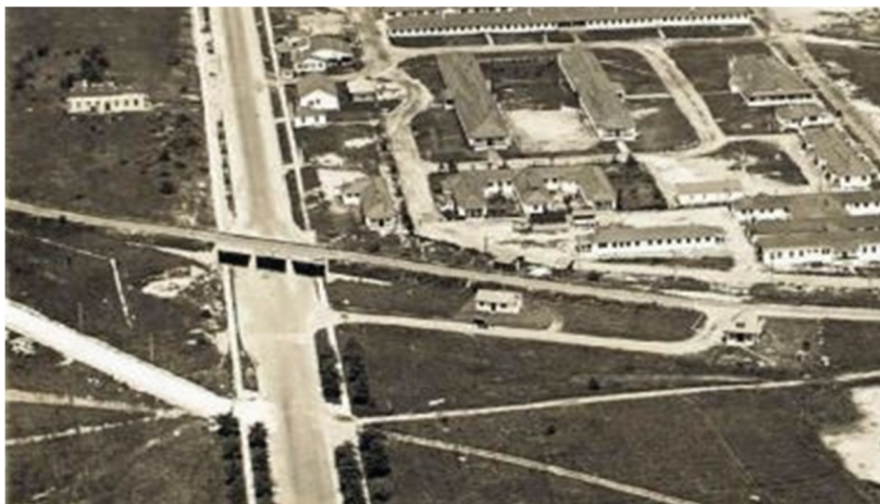
The Motor Parkway bridge over Clinton Rd. with the first Manager's office and Toll Lodge (no porte-cochere yet) at right and airfield buildings upper right
