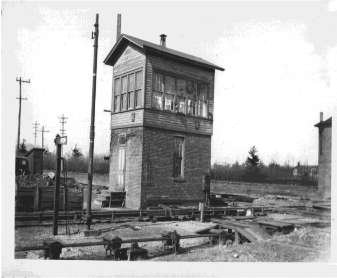
The Wye tower, facing NE.
